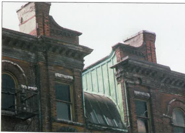
Detail of the skylight. JOHN CONLIN PHOTO
