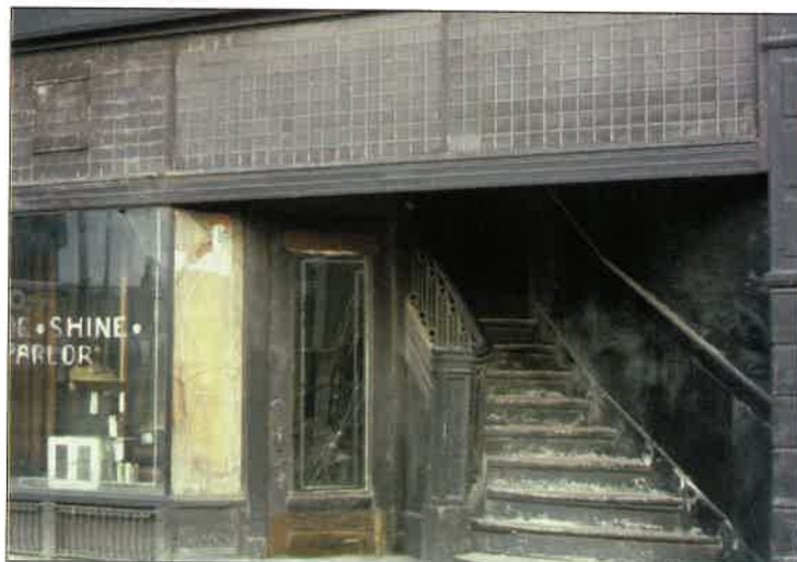
Exterior stairway entrance under "luxfer" transom. JOHN CONLIN PHOTO
