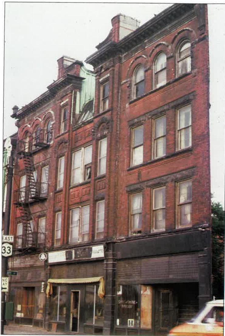
The sharp edge of the facade makes it appear to be free-standing. JOHN CONLIN PHOTO 1980
