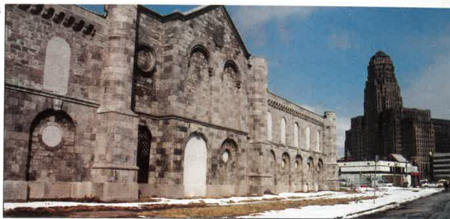
Buffalo Gas Works façade, West Genesee Street, with City Hall in background.
