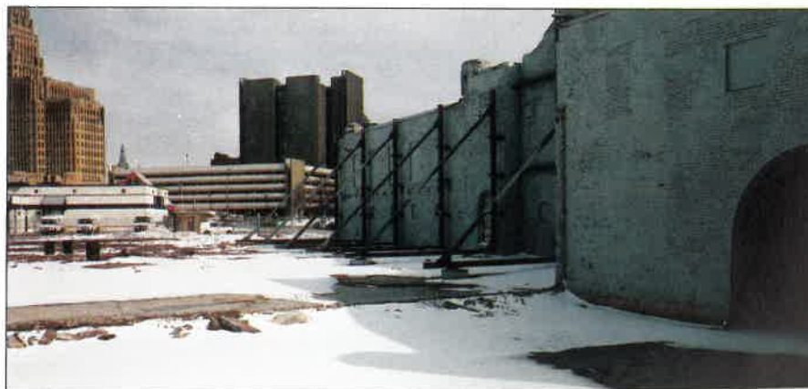
The Hollywood movie set type bracing holding up the façade of the Buffalo Gas Works.
