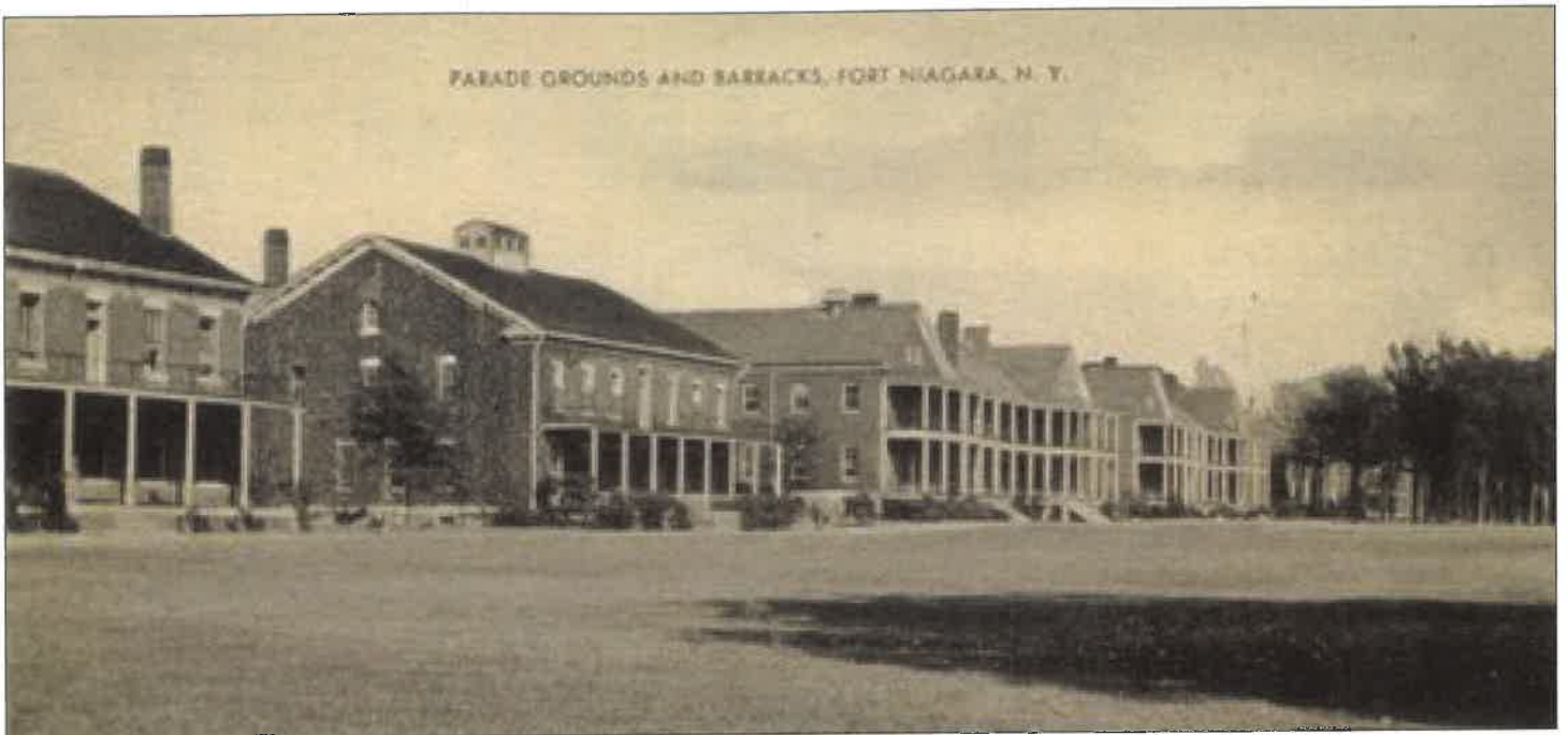
ABOVE: The lineup of barracks buildings at Fort Niagara, c. 1930s. Building 88 is located just into the oak grove in the far distance. PRIVATE COLLECTION
