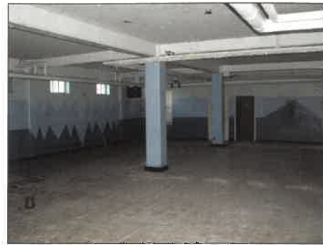
The northwestern dining room in the basement of the barracks. A portion of one of the kitchens is just visible through the door at the rear. The wall paint dates from the building's use by the Young Adult Conservation Corps. COURTESY NYSOPRHP, DOUGLAS W. DeCROIX PHOTO
